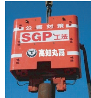
杭打機本体 防音防振カバー取付 Vibrodriver (noise-proof vibration-proof cover installation)
