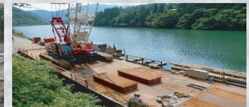
岐阜県：市道林～丸山線災害復旧工事 Gifu/road disaster restoration work
