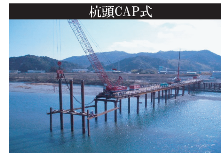
Pile Head Cap Method
