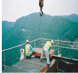
⑧ 覆工板 地覆設置 constructing covering plate
