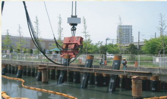
斜杭施工可能 Can construct oblique piles
