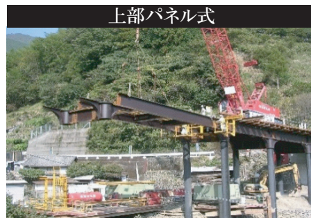
Top Panel Preceded Construction Method
