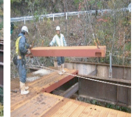
⑦ 覆工板設置 constructing covering plate
