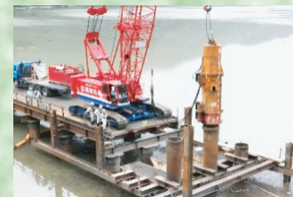
栈橋支持鋼管杭打設 Pier support pile installation
