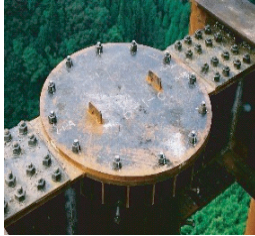
⑦ 杭頭部天蓋取付 mounting pile head canopy
