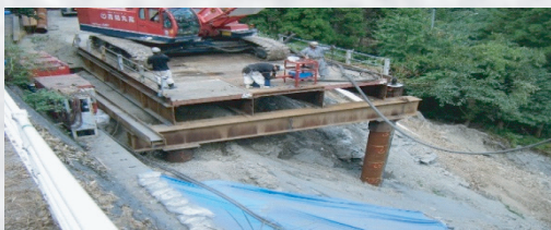
愛媛県：大保木災害道路復旧工事 Ehime/Ofuki disaster road restoration work
