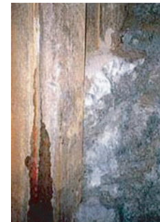
鋼矢板硬岩貫入状況 Steel sheet pile hard rock intrusion situation
