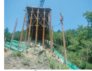
① 導材設置 constructing guide members
