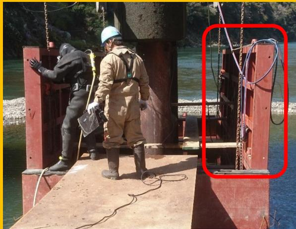
鋼管補強当板：巾441.5mm、厚み  $t = 10\text{mm}$
